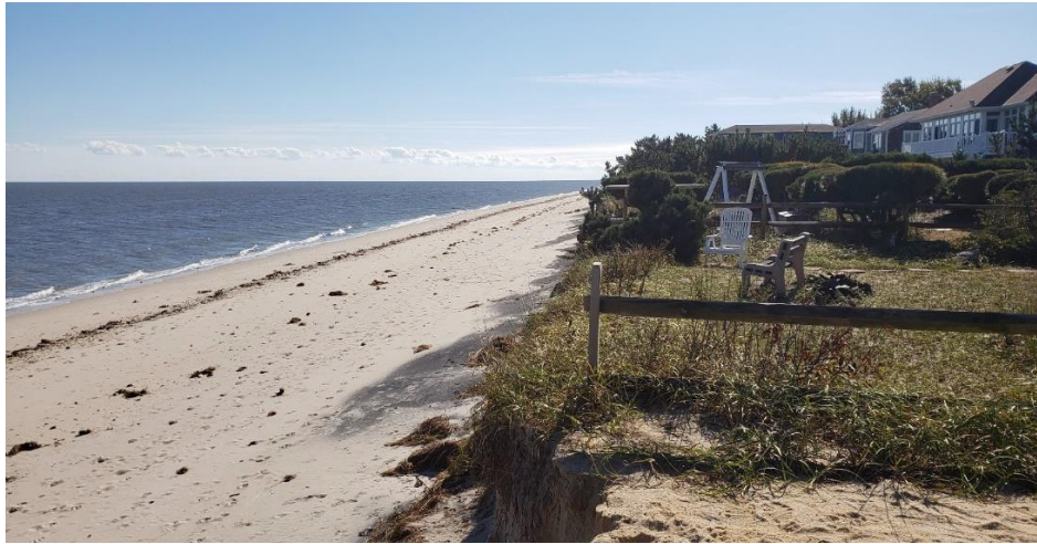
Figure 21: Severe erosion creating an unstable, vertical scarp in Slaughter Beach
