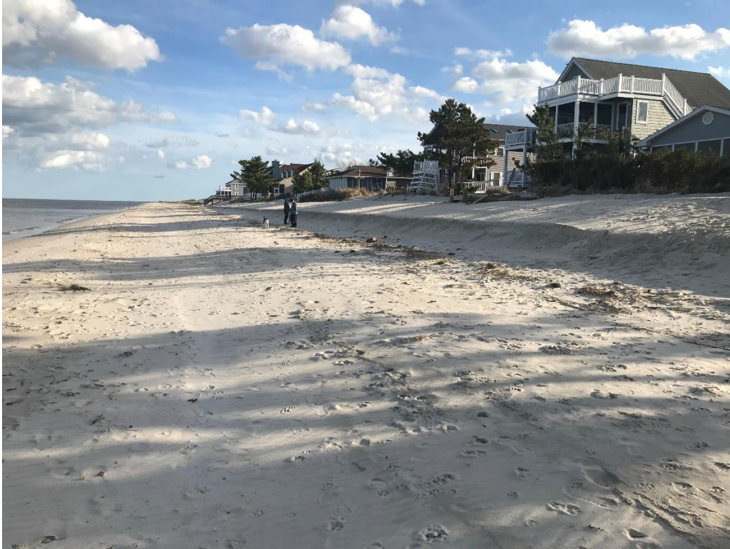
Figure 22: Slaughter after completion of the February 2022 nourishment job. The lower part of the steep template was reshaped into a relatively flat berm.
