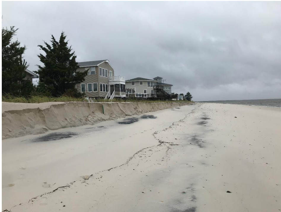
Figure 38 Pickering Beach conditions in October of 2022 which depicts the erosion of the beach fill project completed in April of 2022.
