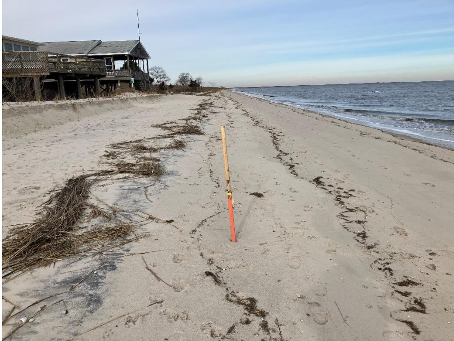
Figure 38 Conditions at Pickering Beach following a December 2022 storm that partially eroded the smaller beach fill job completed in November of 2022.
