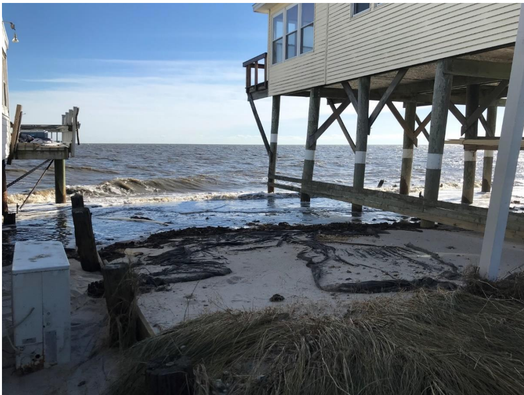
Figure 38 High tide reaching the pilings of homes in Pickering Beach
