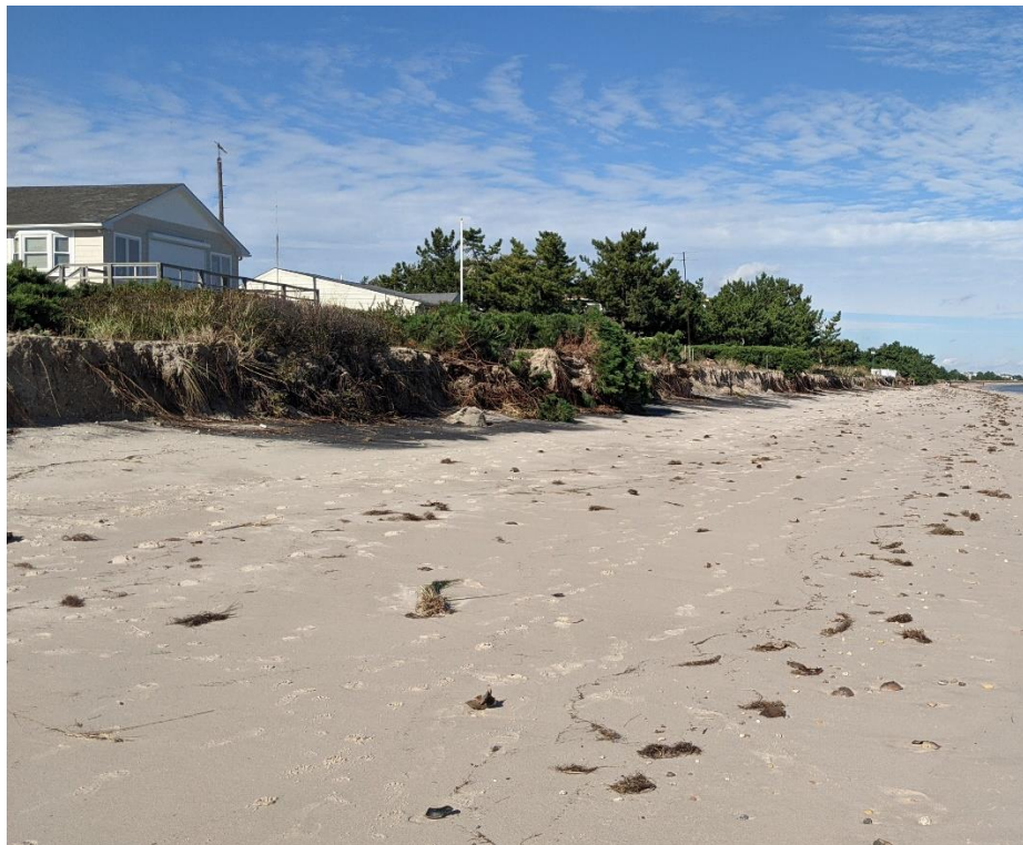
Figure 15: Slaughter Beach bluff erosion during the Fall of 2021. In the southernmost 2000' of the community, from Simpson to Sussex Ave where the bluff encroaches closest to homes.
