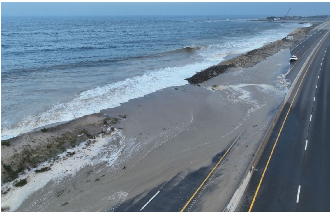
Figure 10E. DE Seashore State Park - North Inlet Beach (8/17/2024) at high tide looking south. The Rt 1 northbound lane is closed as ocean water breaches the dune and floods the roadway.
