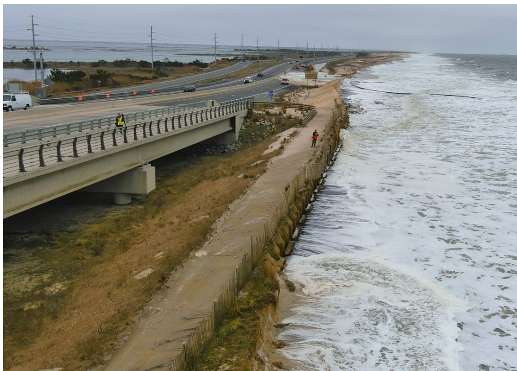
Figure 10D. North Inlet Beach (3/26/2024) at high tide looking north. Ocean water covers the NB Rt 1 lane just beyond the Inlet Bridge, visible on the left.
