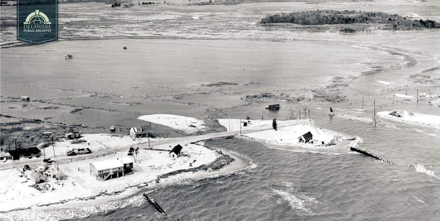
Slaughter Beach storm damage - 1962
