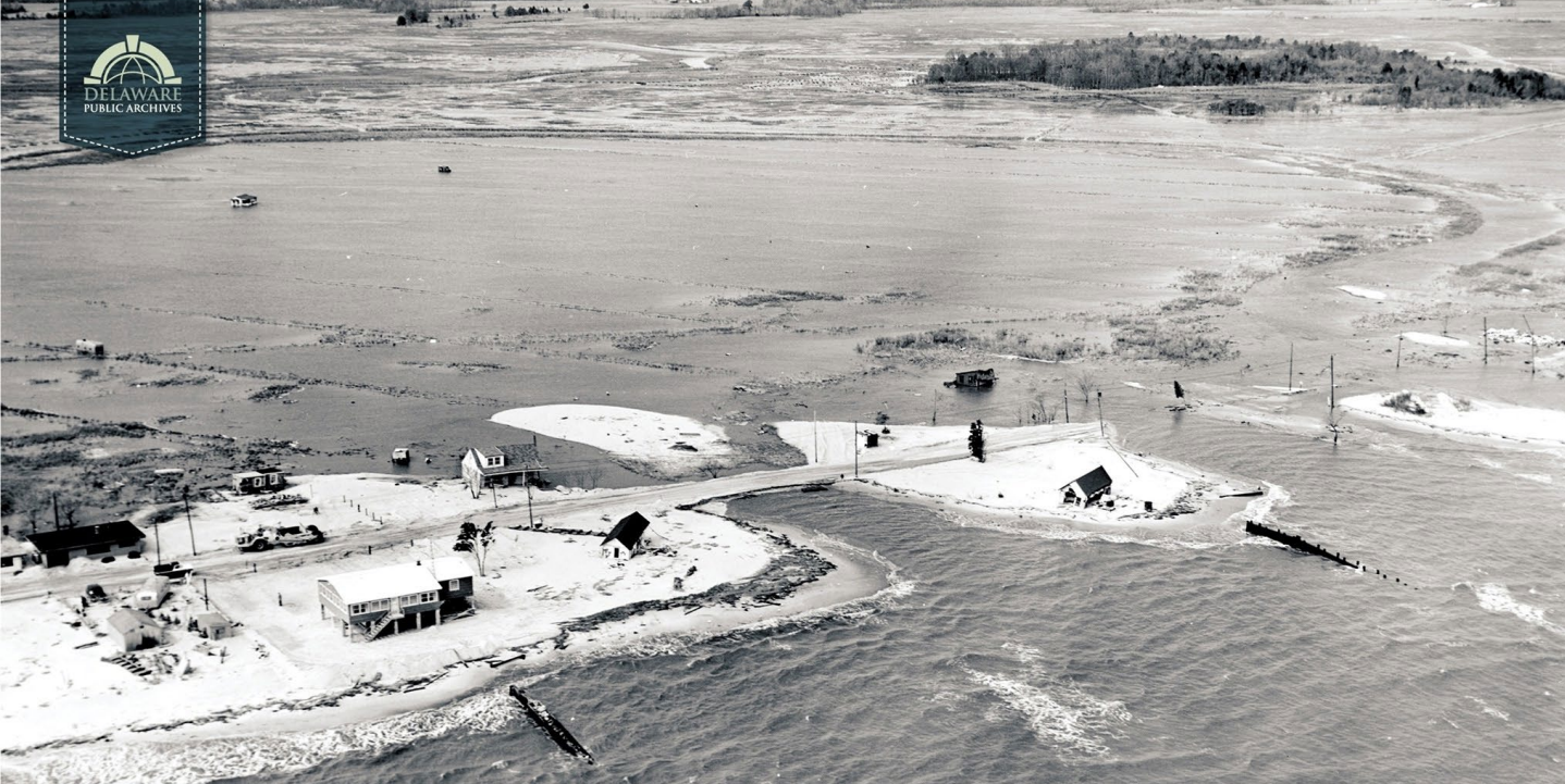
Slaughter Beach storm damage – 1962
