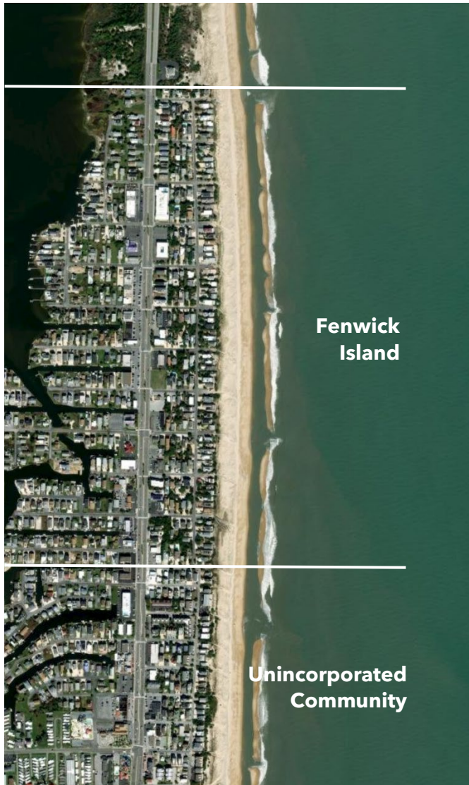
Figure 14-4. Due to sand spreading, nourishment at Fenwick Island results in infrastructure benefits to a community to the south
