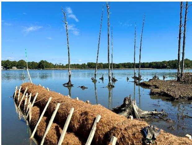
Figure 8. A coastal wetland and shoreline restoration project in Millsboro, Delaware.
