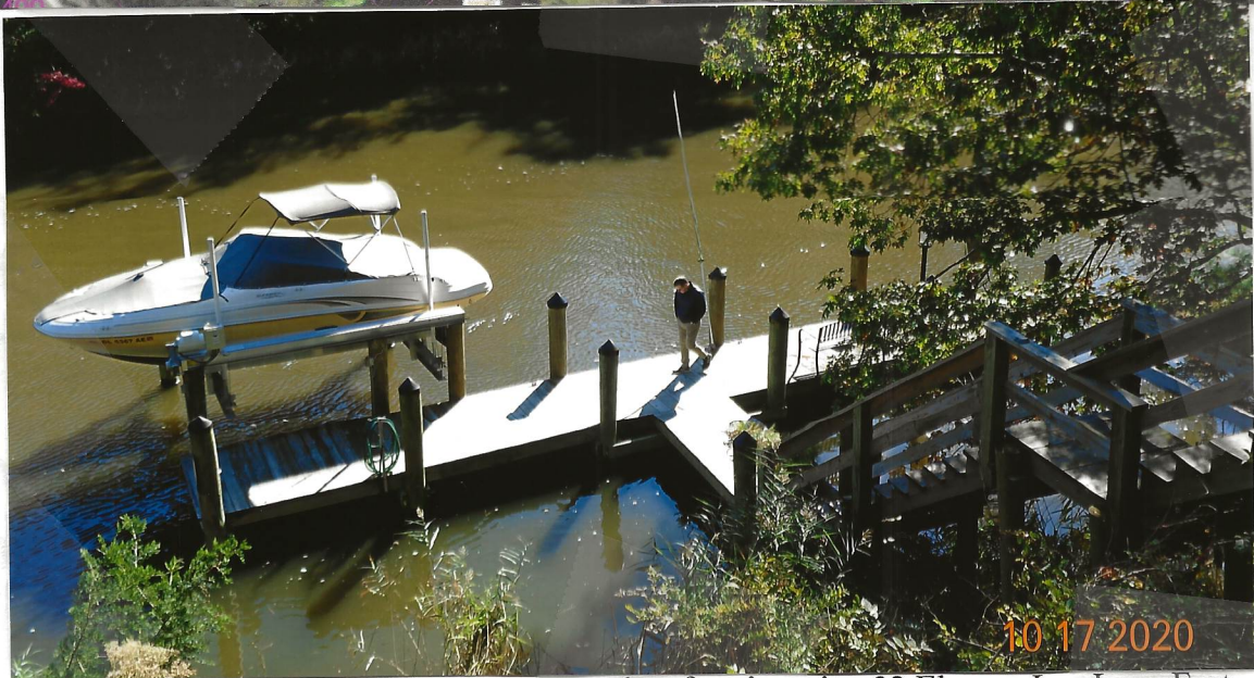
Figure 5. Aerial and ground-level photographs of project site, 32 Eleanor Lee Lane East, Canal Corkran, Rehoboth Beach, Sussex County, Delaware, adjacent to the Lewes and Rehoboth Canal, showing existing structure, 10' x 4' pier and 6' x 45' dock with boat lift (authorized by SP-283/14) and CENAP-OP-R-2014-1200-23). Width of waterway = 120'±. Applicants propose to add a PWC lift (on existing piling), and to install a 6' x 12' floating kayak dock with two support pilings. See Figure 6 for plan view and cross-section sketches.
