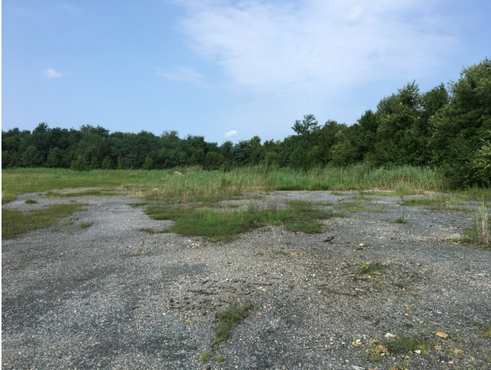
Photograph 2: Overgrown paved areas on the project site.
