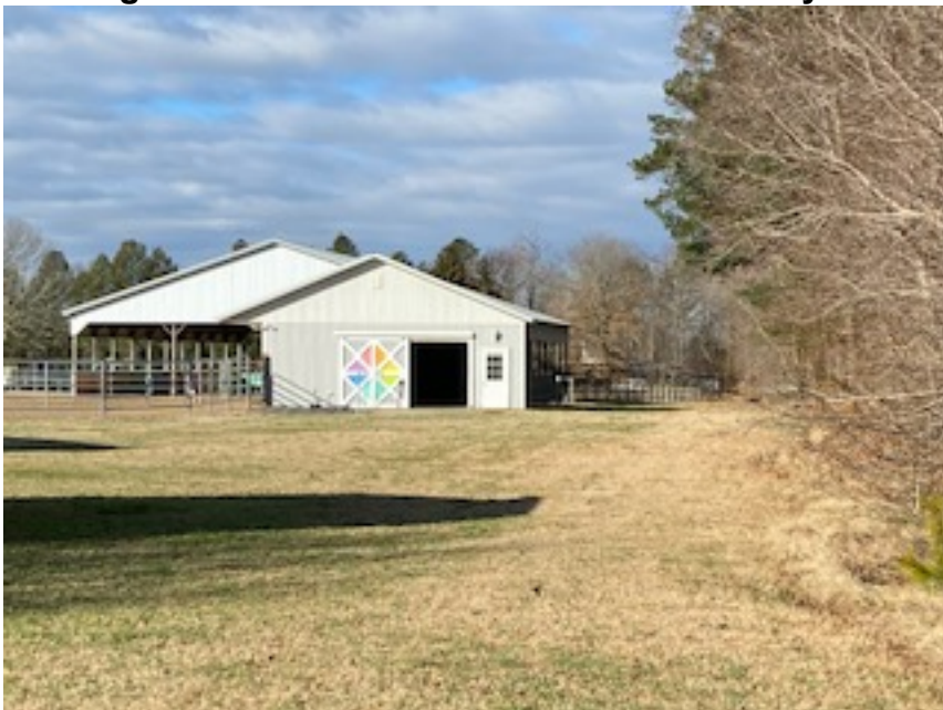
Barns located adjacent to property
