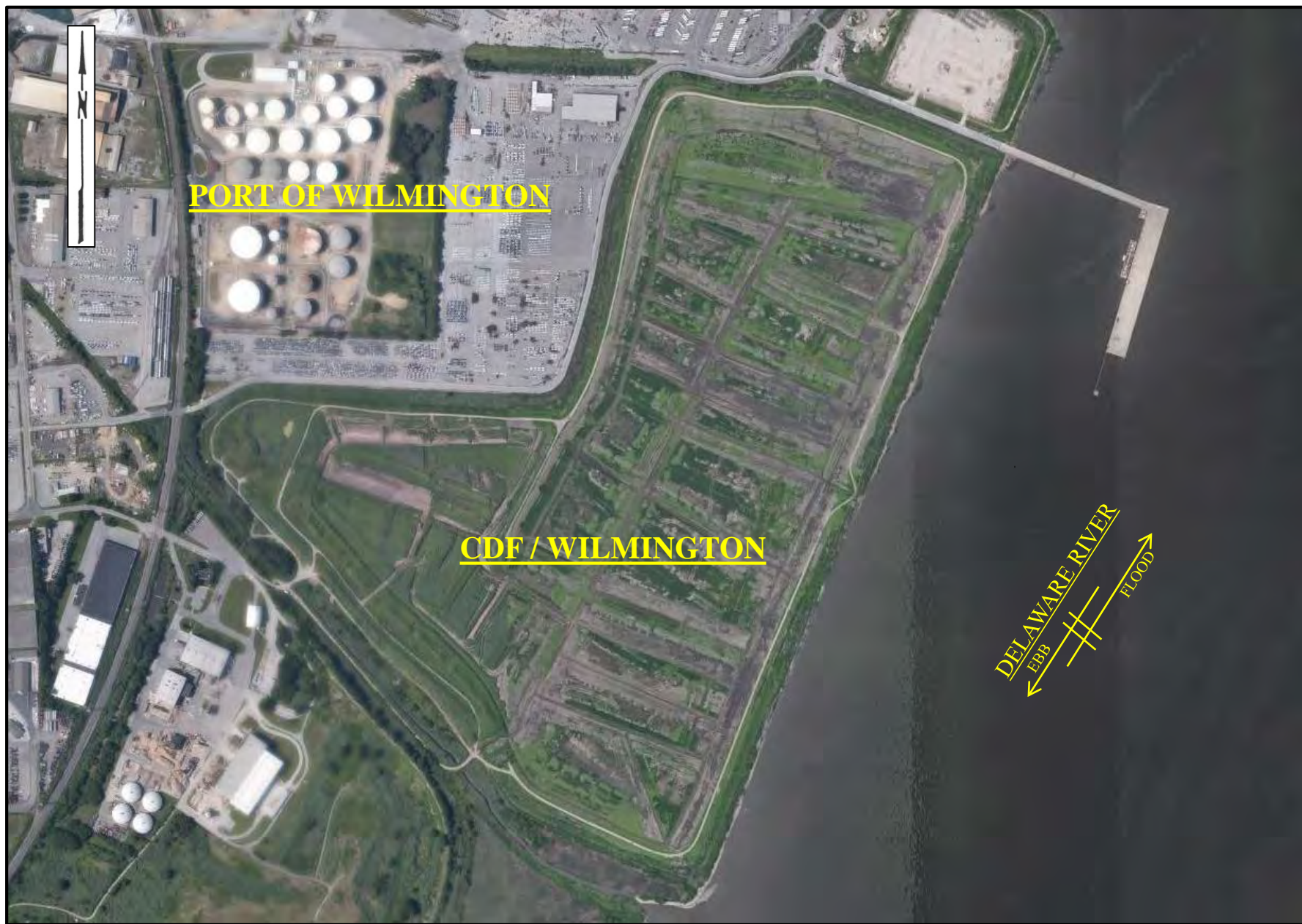
AERIAL PHOTO OF THE WILMINGTON HARBOR SOUTH CONFINED DISPOSAL FACILITY
