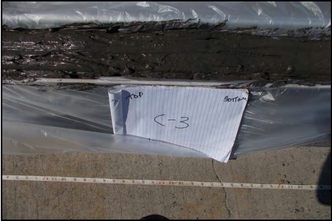
PHOTO No. 11: C-3, CENTER
