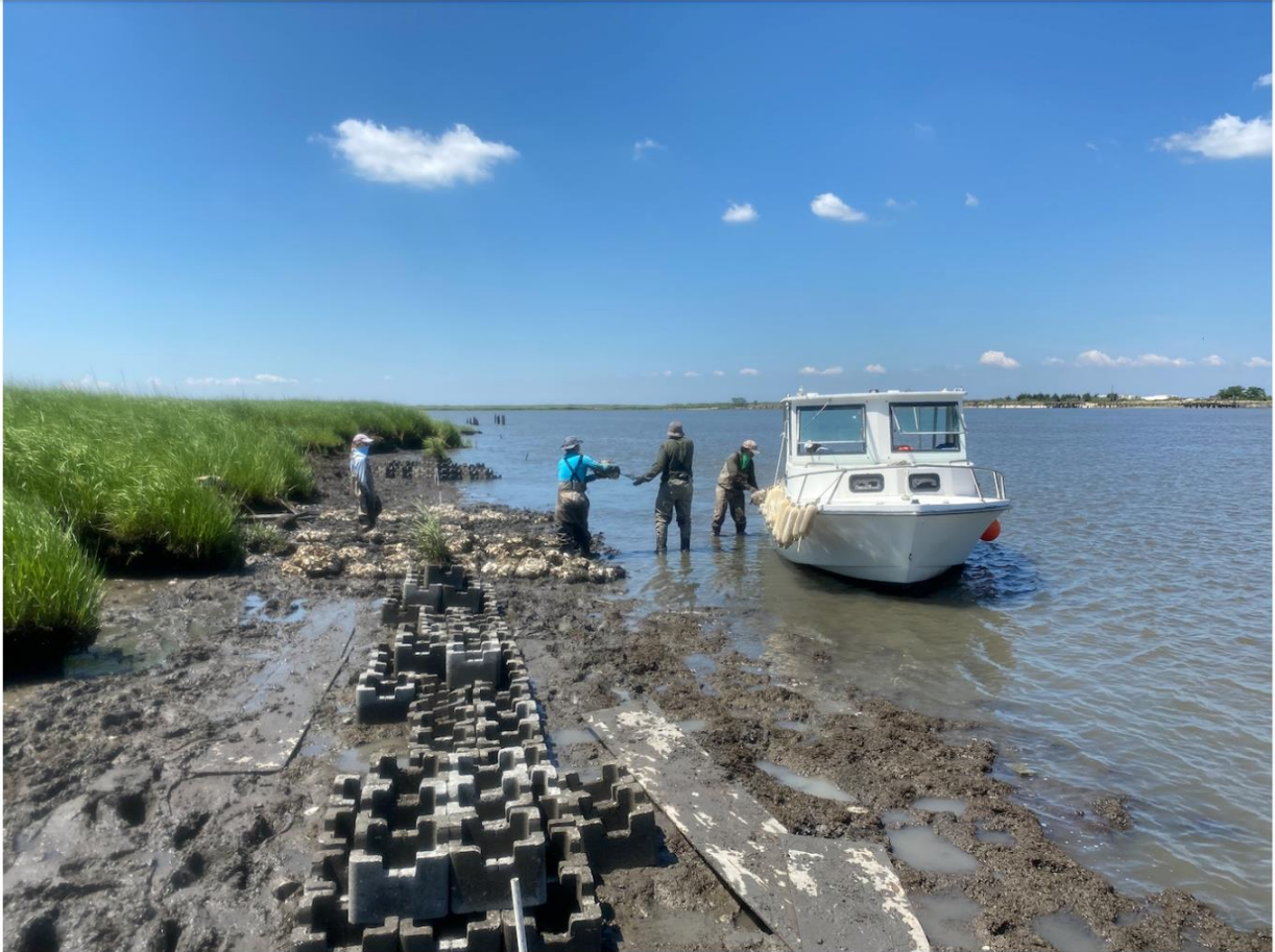
Figure 13: DELSI Maurice River oyster castles and oyster shell bags 2020 living shoreline project (photo courtesy of D. Bushek, Rutgers University Haskin Research Lab).
