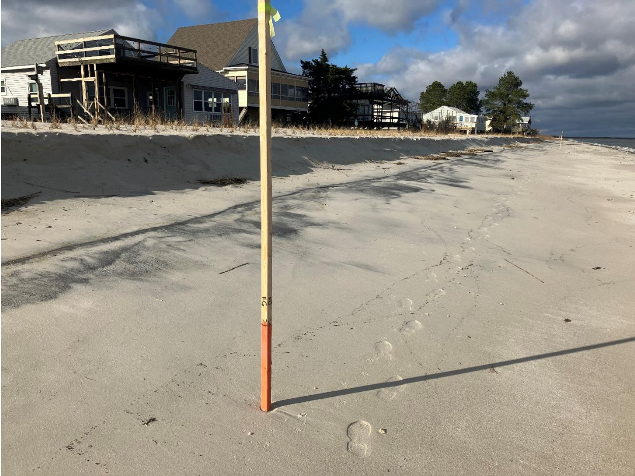
Pickering Beach 12-23-2022 after a fall replenishment project, coastal storm eroded beach to pre-fill template.
