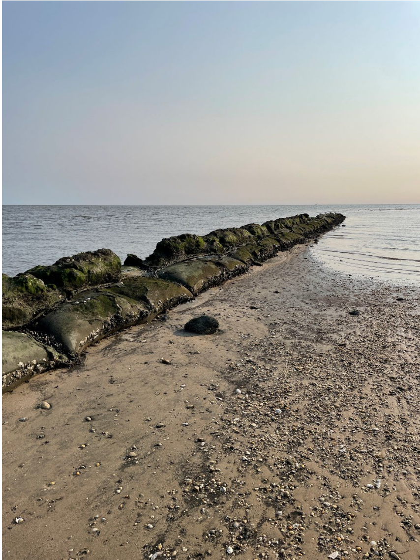
Northeasterly view of the seaward end of the south jetty.
