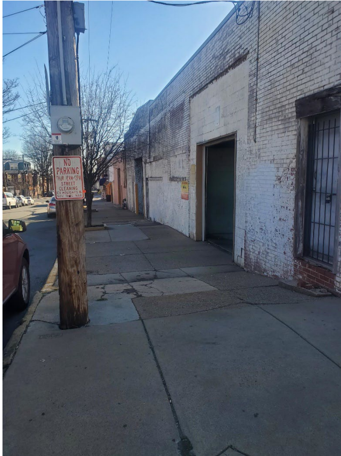
Sidewalk/entry to all three garages from 5 th Street
