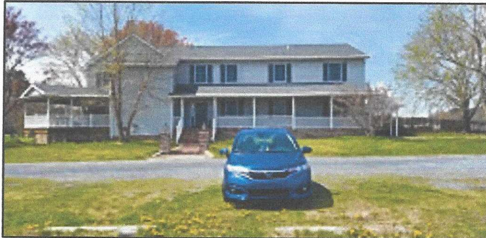
Photograph No. 2 Shawnee Inn (View looking Southwest) 11116 Shawnee Road 19958 - Tax Parcel No. 430-3.00-6.02
