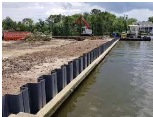
Example of newly installed bulkheading.
