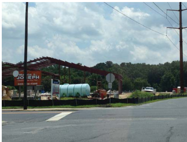
The view of the site from across Clayton Street looking southeast.
