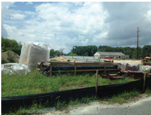
Looking northwest from Lingo Road onto the site.
