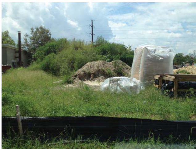
A dirt mound with large weeds sits on the eastern corner of the site and tall weeds line Lingo Road, which runs northeast of the site.
