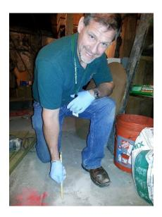
4) Use drill bit to penetrate through any sub-slab material (1" or 2.5 cm) to create an open cavity in order to prevent potential obstruction of probes during sampling.
