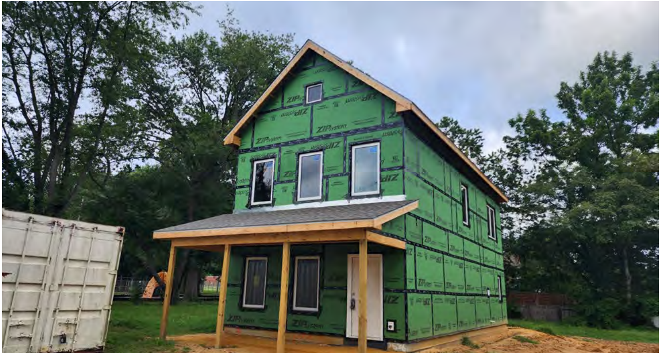
Passive house under construction in Dover, featuring a continuous air barrier system to reduce air leakage. PHOTO: JESSICA QUINN, DNREC
