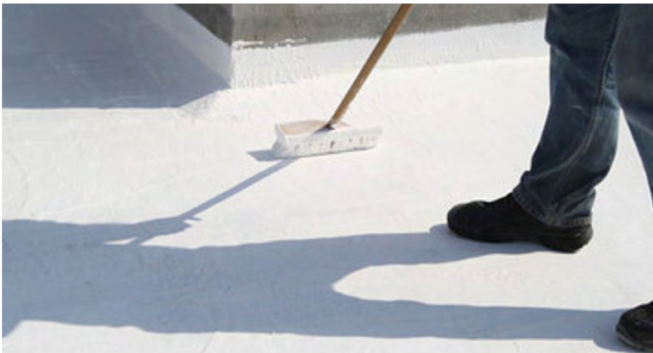
White roof coatings reflect sunlight and reduce heat absorption, lowering indoor temperatures and supporting climate resilience. PHOTO: ADOBE STOCK
