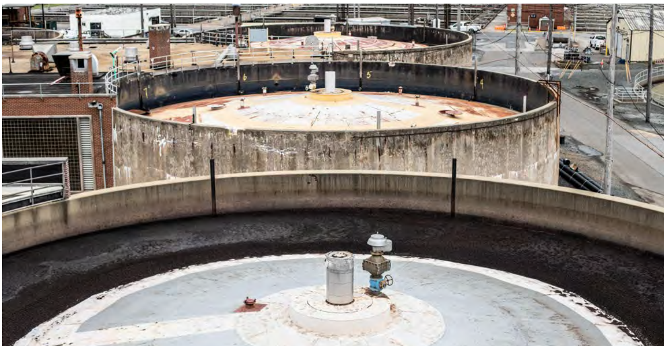
Digester tank covers at the Wilmington Wastewater Treatment Plant. PHOTO: CITY OF WILMINGTON
