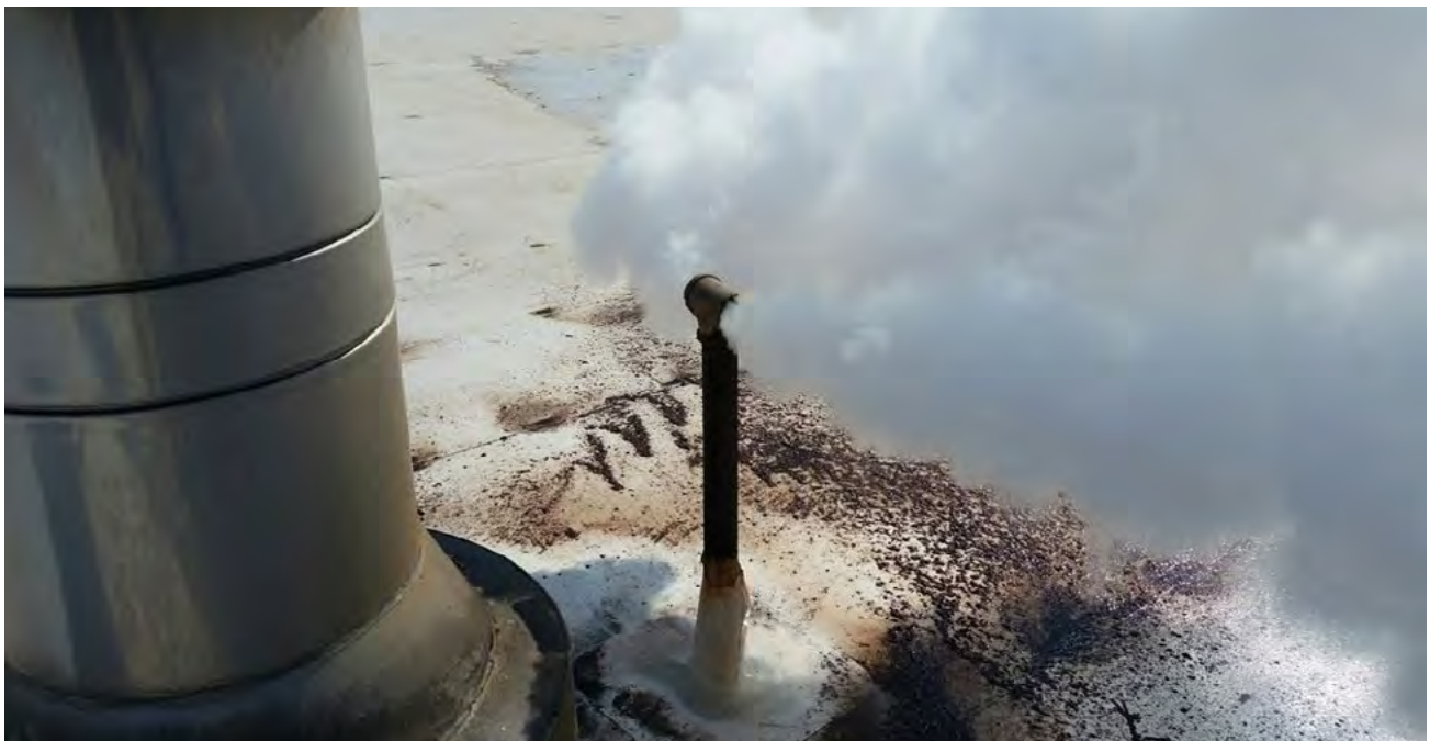
Extreme flash steam occurring at a power plant. Flash steam recovery is a common energy efficiency measure in industrial settings. Recovery of the flash steam at this site as hot water for the plant's processing systems saves over $10,000/year in natural gas costs. PHOTO: UNIVERSITY OF DELAWARE
