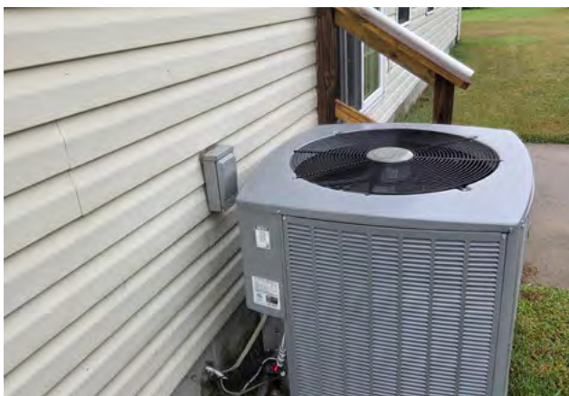
Residential heat pump. PHOTO: DNREC
