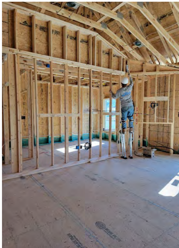
Worker installing air sealing foam to reduce air leaks, increasing energy efficiency and occupant comfort. PHOTO: DNREC
