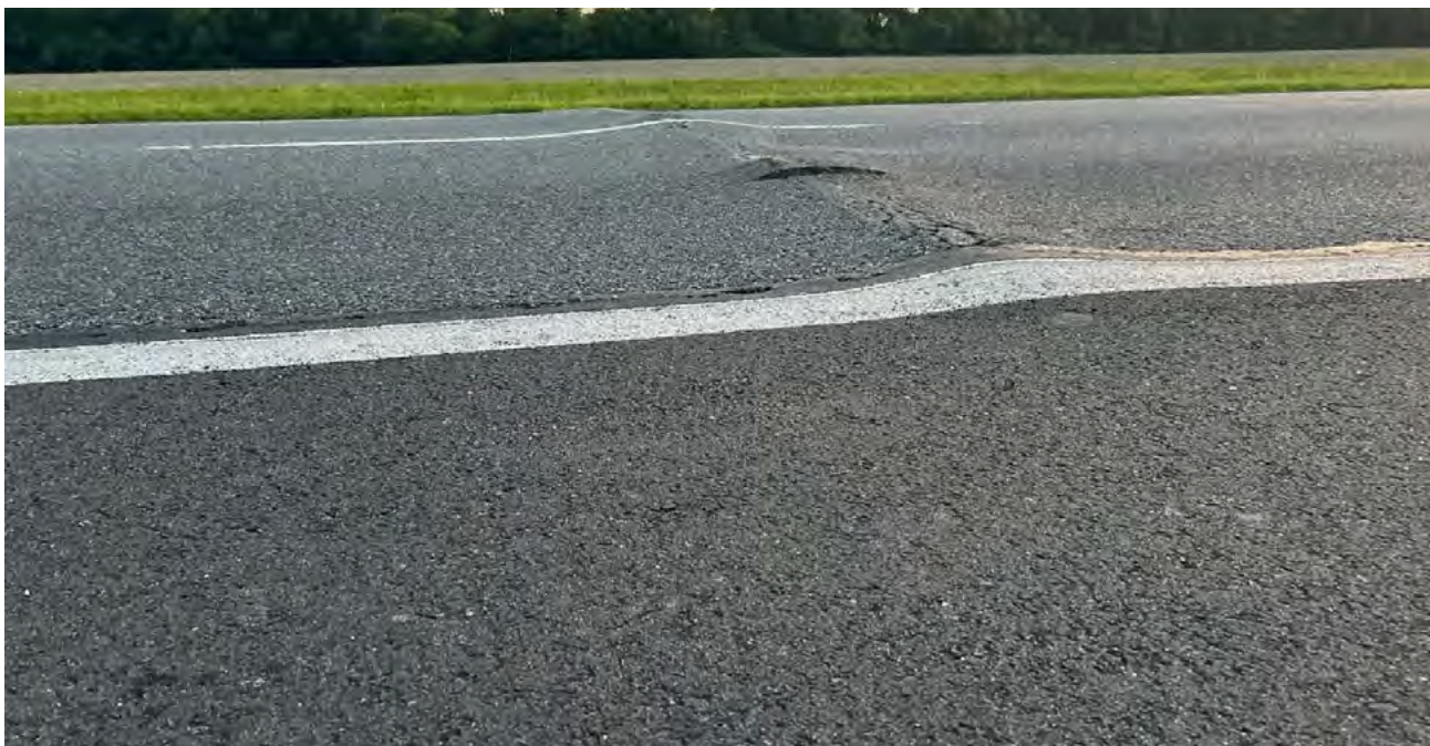
An intense heat wave in June 2025 caused Delaware roads to buckle. PHOTO: DELDOT
