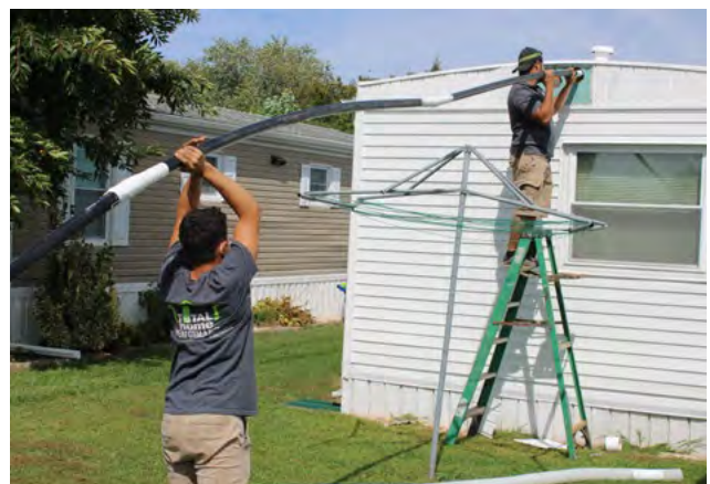
Weatherization Assistance Program contractors installing insulation. PHOTO: DNREC
