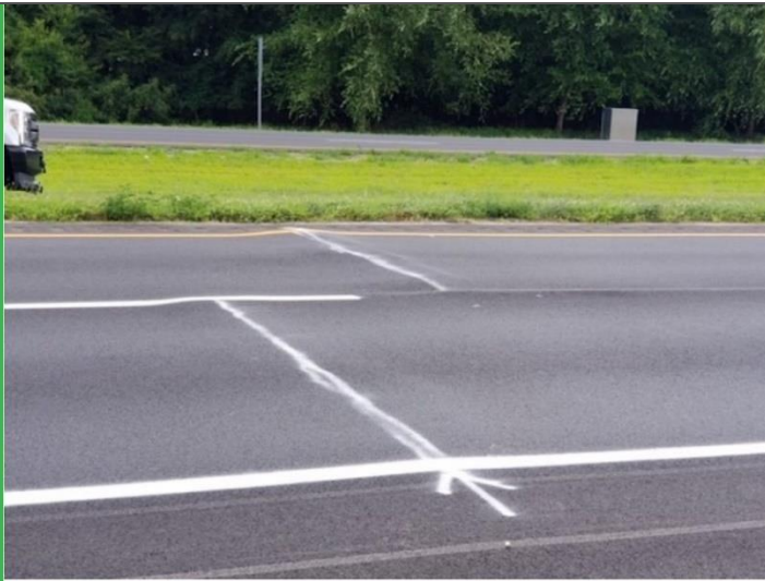
A section of Delaware Route 1 near Milford was damaged by a “road heaving” incident that caused the roadway to buckle. Asphalt surfaces and other materials can be damaged during heat waves.
