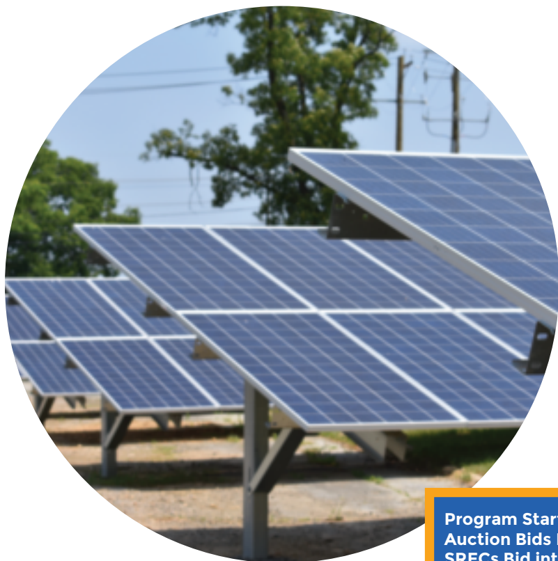
Solar panel system
