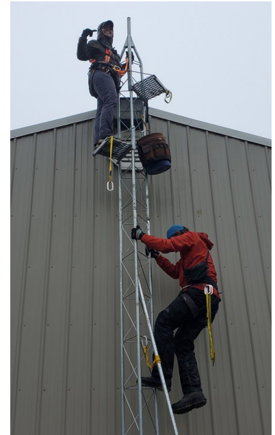
Motus tower install
