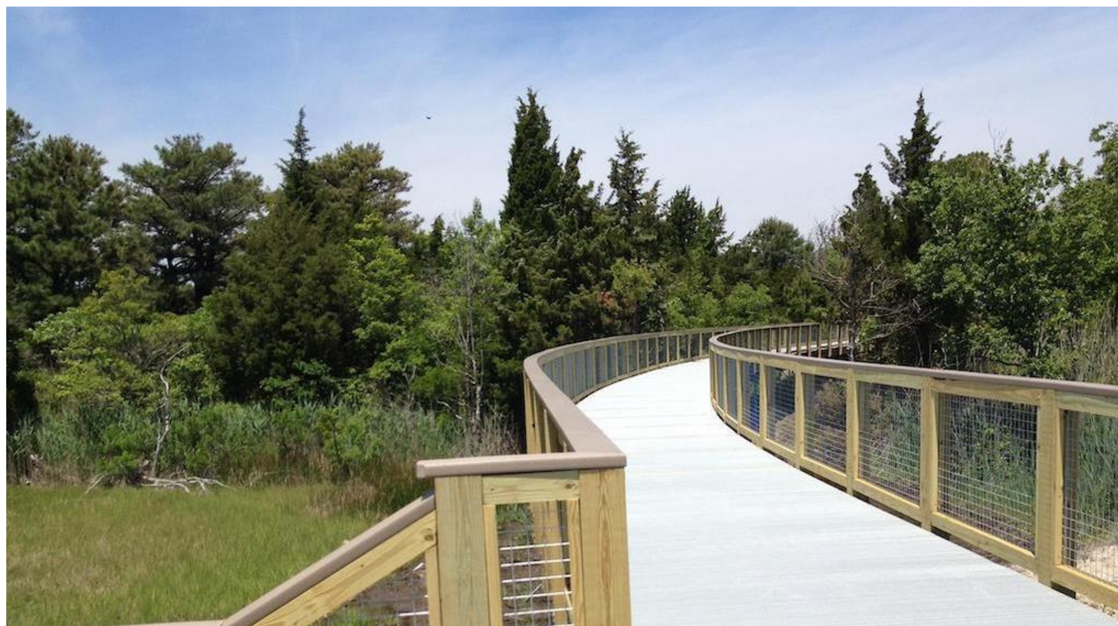
Example of an 8' wide raised trail section at Gordon's Pond trail. Image courtesy of Rails To Trails Conservancy.
