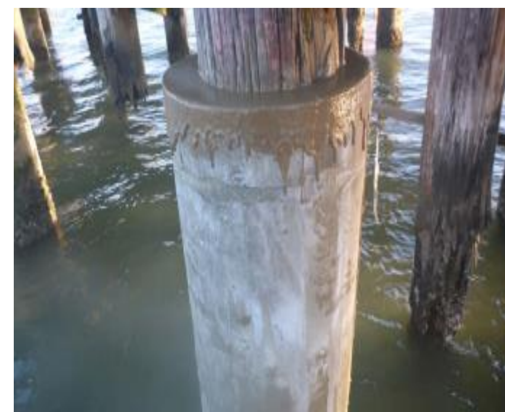
After Fiberglass Jacket
