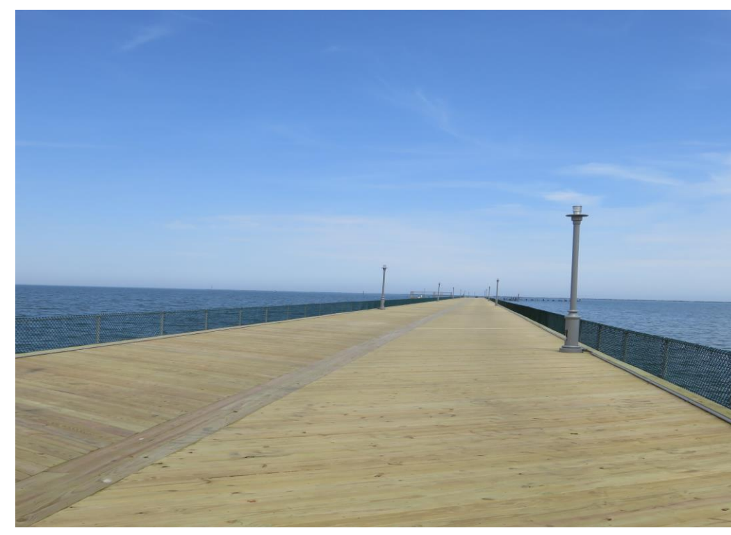
After Deck Replacement
