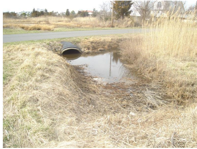
Figure D.30: Ditch crossing Market St. 600 ft. north of Anglers Rd. with evidence of water flowing from canal into the Market St. ditch system (LB_03)
