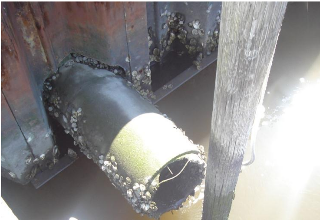
Figure D.31: The existing Savannah Rd. storm drain conveyance system outfalls to a 24 inch concrete pipe that is below the high water elevation (LB_04)
