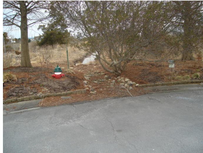
Figure D.28: Stone outfall from Rehoboth Cul-de-sac to the ditch that runs parallel to Cedar Ave. (LB_01)
