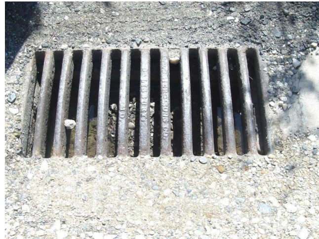
Figure D.32: Grate inlet full of debris in the alley south of Market St. (LB_14)
