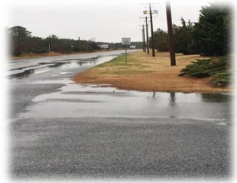
Existing pavement sump located between the edge of pave and driveway entrance
