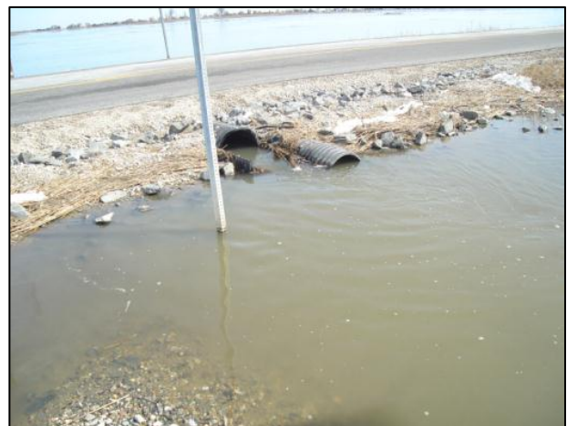
Sedimentation and existing storm drain pipes at Prime Hook Road (PH_11)
