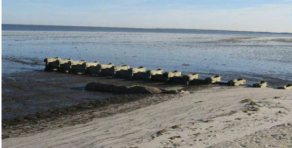
Figure 7.15 Terminal groin and an outfall structure at the south end of Kitts Hummock.
