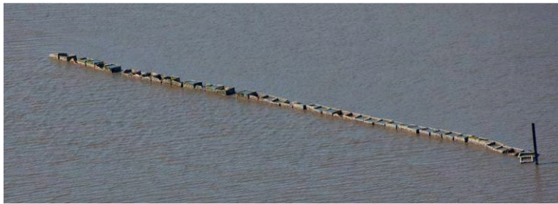
Figure 7.13 Concrete box breakwater constructed by the Corps in 1979 (Wayne Lasch, April 17, 2009).
