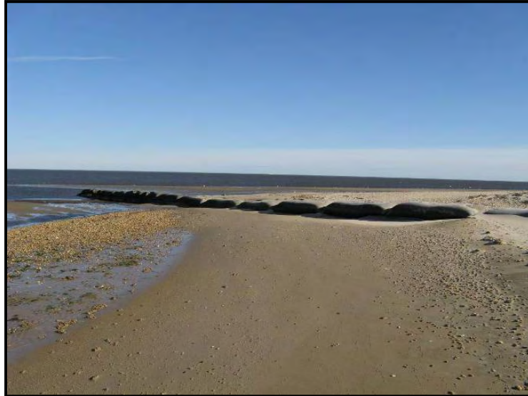
Figure 7.23 North terminal sandbag groin.
